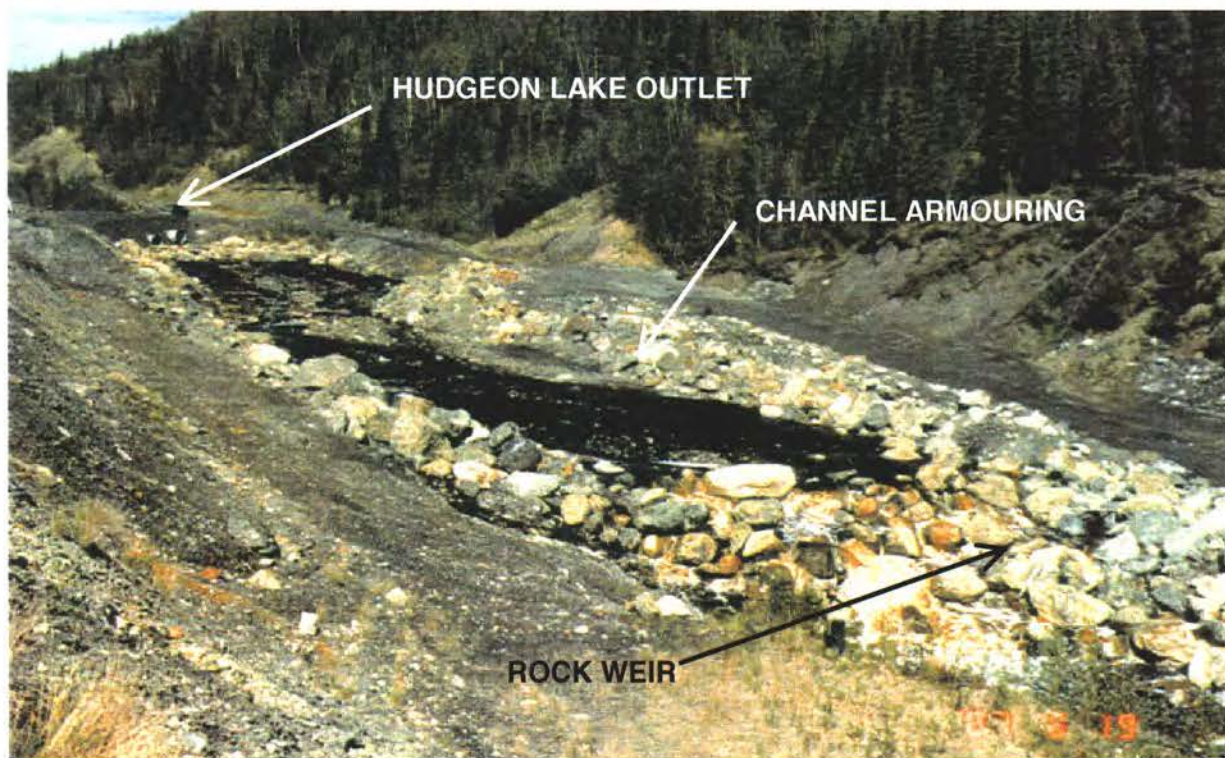
Photo 5 Rock Weir and Channel Armouring
