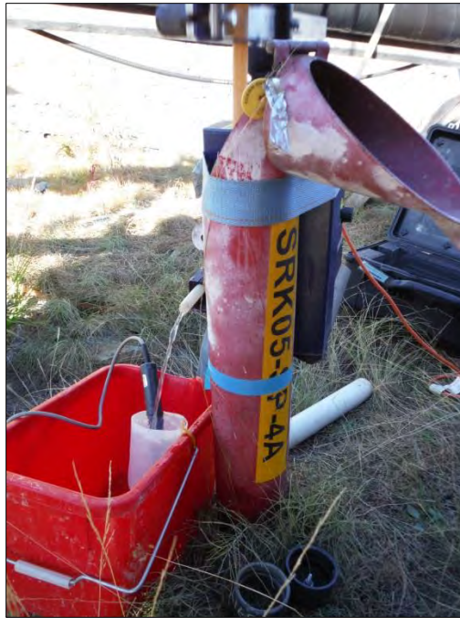
Photo 51: View of well SRK05-SP-4A. Photo taken on September 9 th , 2014.
