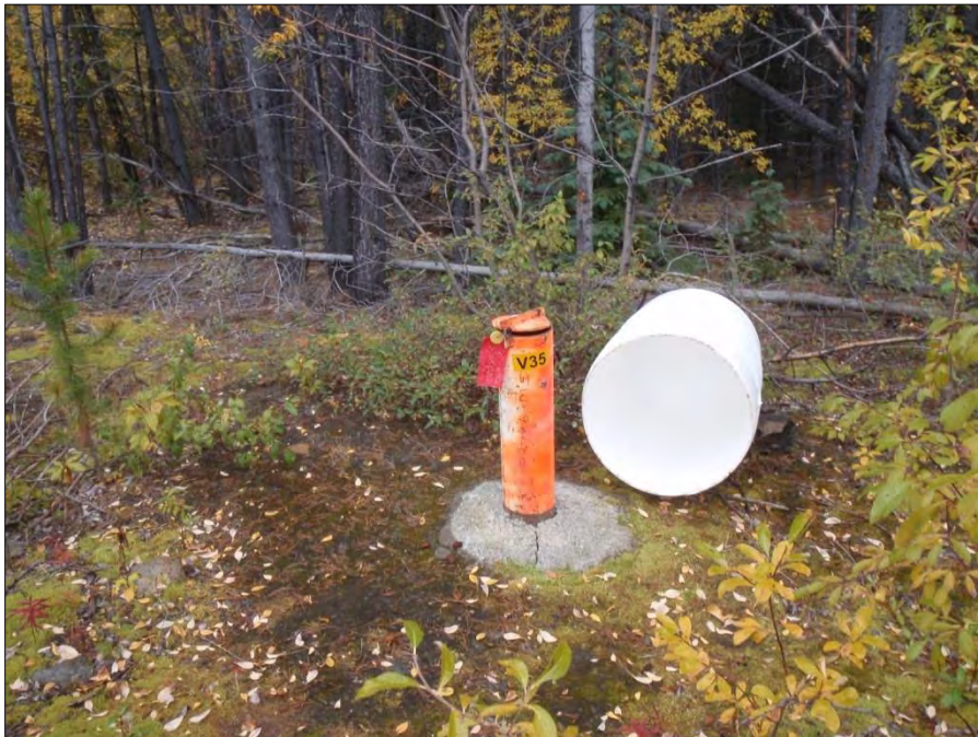
Photo 88: View of well V35. Photo taken on September 11 th , 2014.
