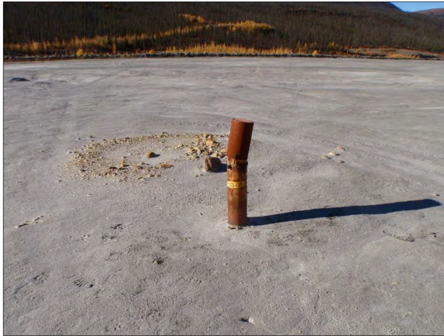
Photo 39: View of well P03-05-4. Photo taken on September 15 th , 2014.
