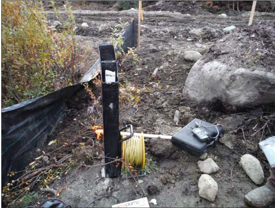
Photo 65: View of well MW14-11. Photo taken on September 10 th , 2014.
