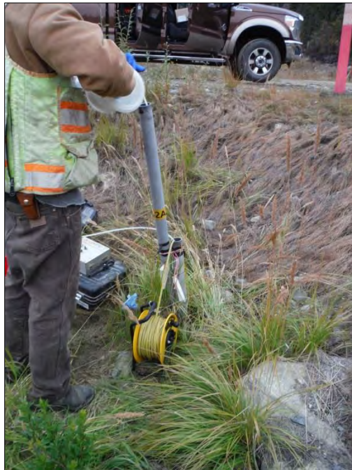
Photo 48: View of wells S2A and S2B. Photo taken on September 10 th , 2014.
