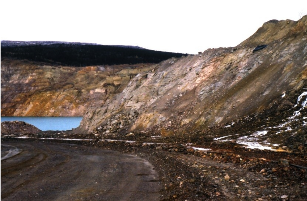
Looking upstream along toe of left abutment.
