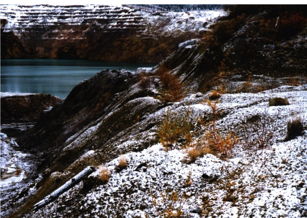
Looking upstream along top of left abutment. Diversion ditch and berm on bench.
