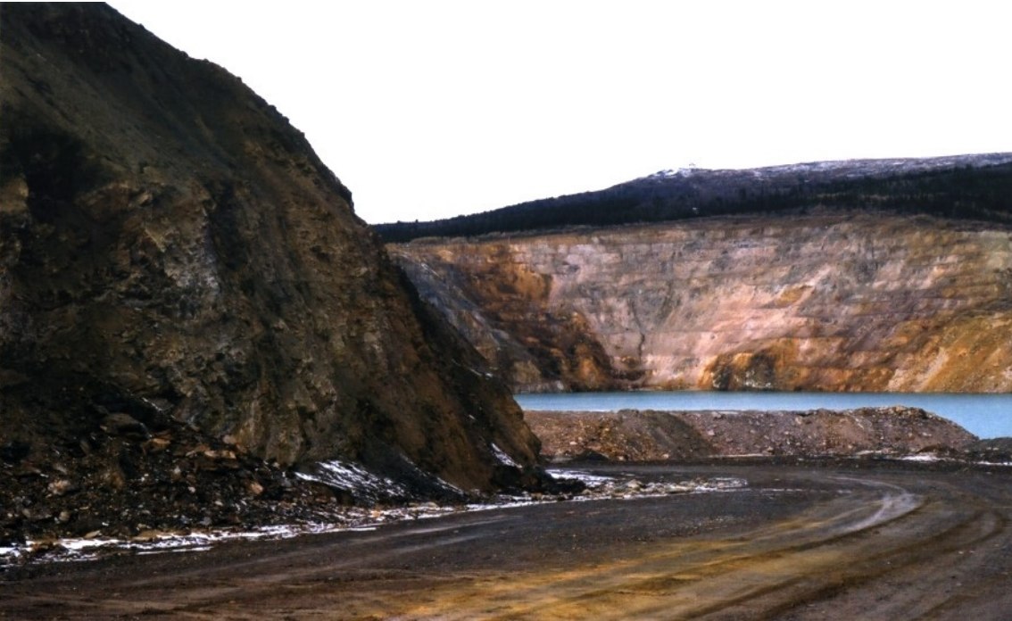
Looking upstream along toe of right abutment.
