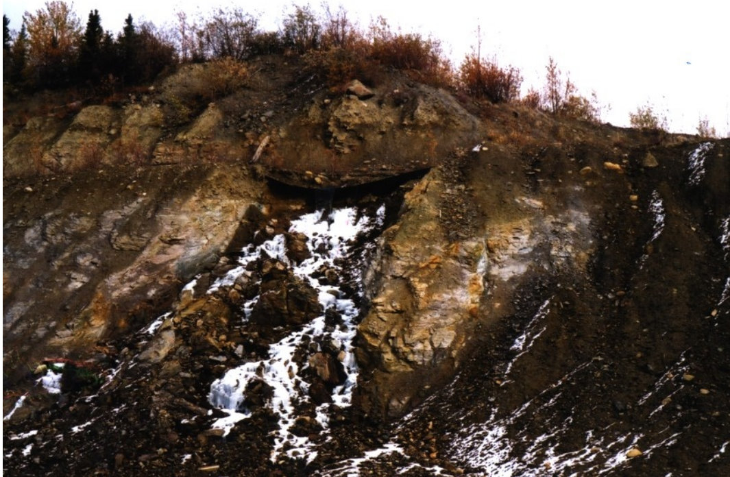
Small - scale wedge failure in left abutment has breached diversion ditch and liner on upper bench
