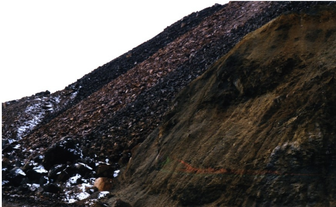
Edge of bedrock on right abutment at edge fo Zone II pit filled with waste rock.
