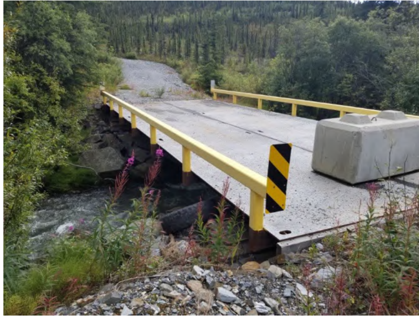
Photo 6 - Lightning Creek Bridge Abutments, Onek Road (August 18/20)
