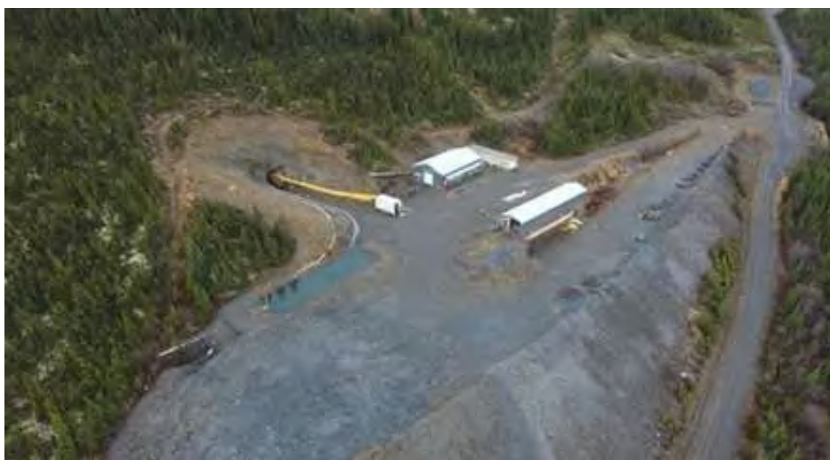
Photo 2-2: Lucky Queen Surface View from 2018.
