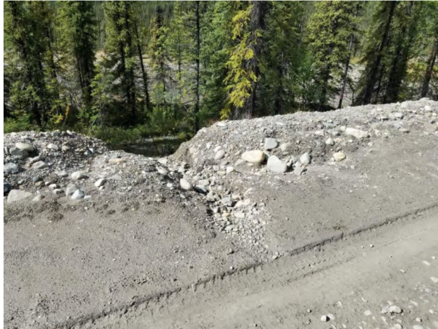
Photo 8 - Mill Storage Ponds, Access Road Erosion (August 18/20)
