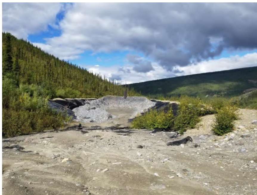
Photo 1 - Bellekeno PAG Storage Facility (August 18/20)
