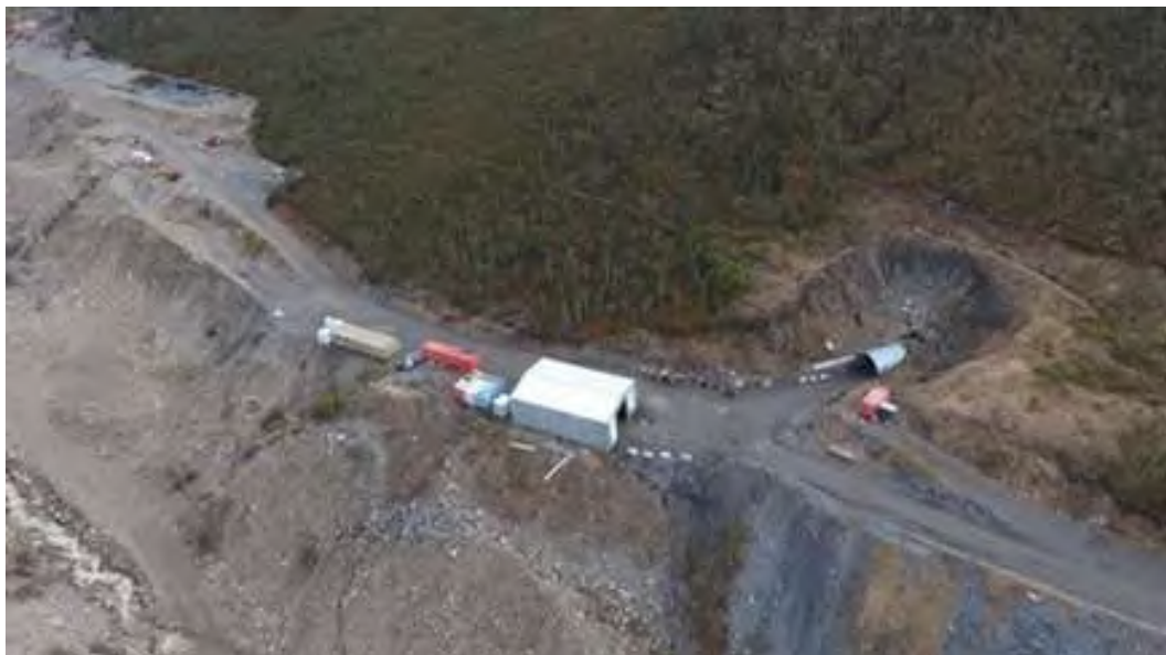
Photo 2-1: Bellekeno East Portal and Surface Facilities from 2018. Note shop was removed in 2020.
