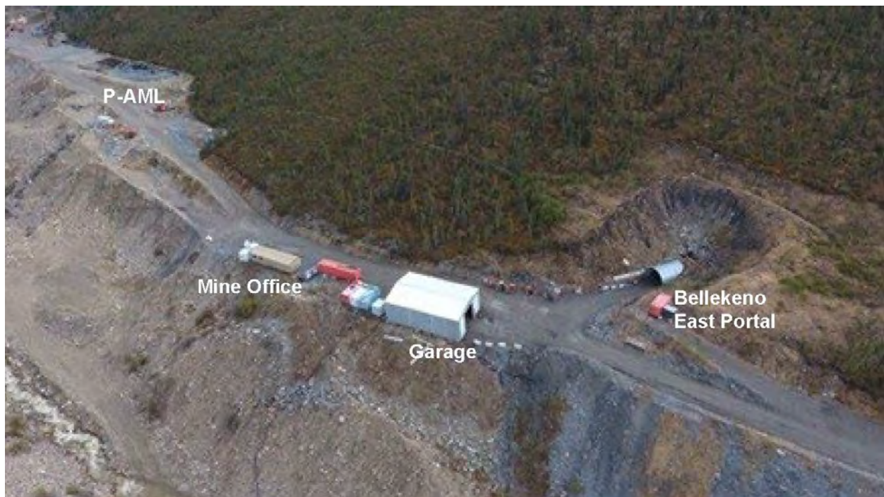
Photo 2-1: Bellekeno East Portal Surface Facilities from 2018.
