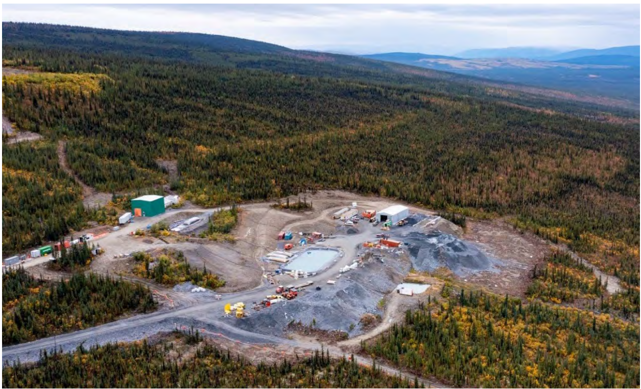
Photo 2-3: Bermingham Surface View from September 2021.
