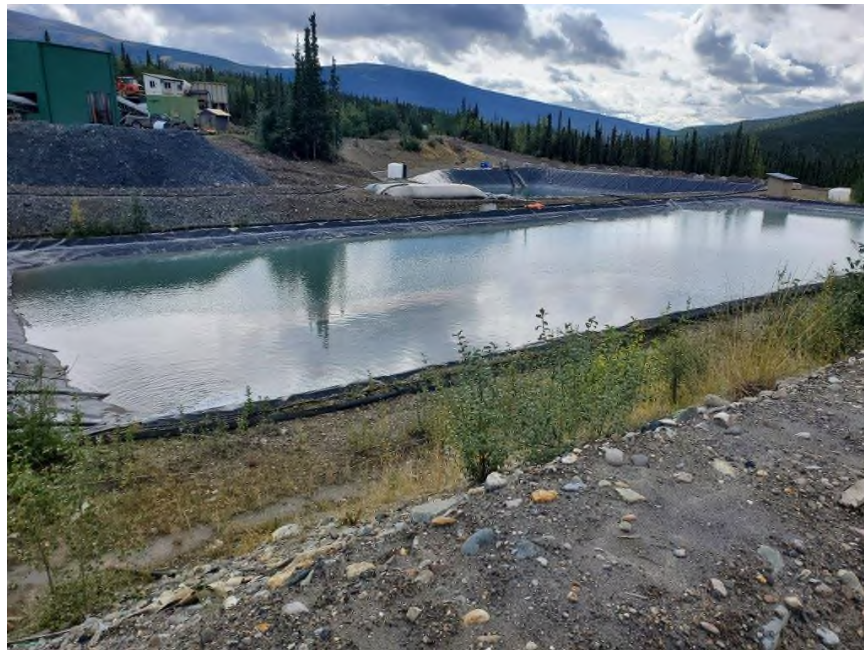
Photo 7: Mill Water Storage Pond (August 26/21)
