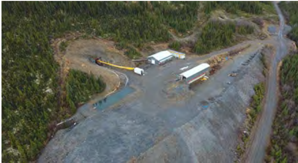
Photo 2-5: Lucky Queen Surface View from 2018.
