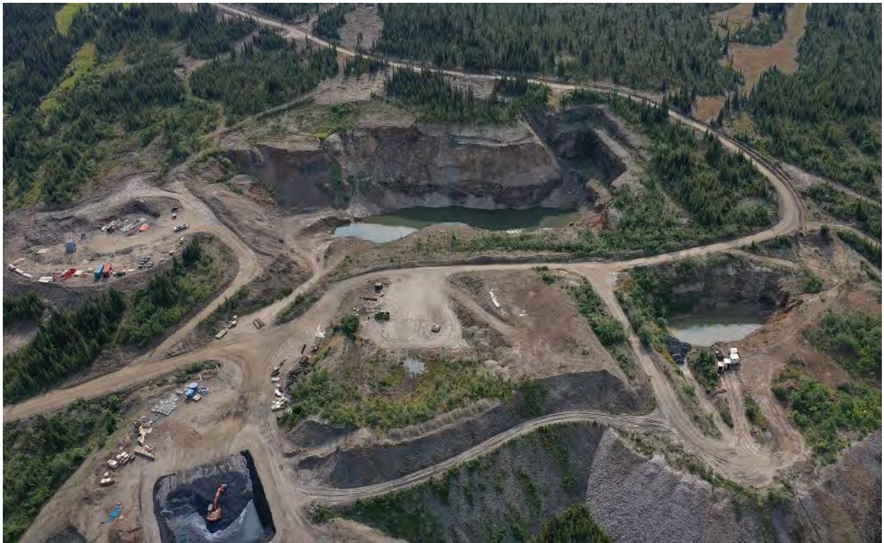
Photo 2-4: Bermingham Vent Raise View from August 2021.
