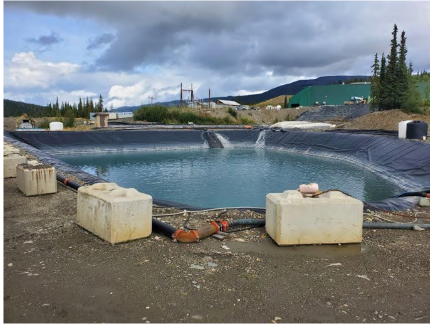
Photo 8: Mill Water Storage Pond (August 26/21)
