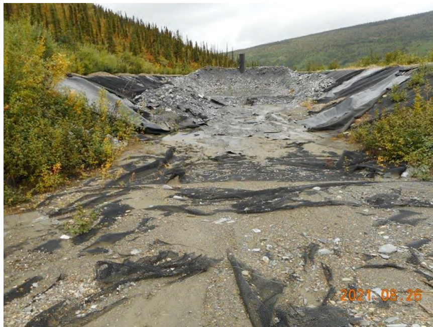
Photo 1: Bellekeno PAG Storage Facility (August 26/21)
