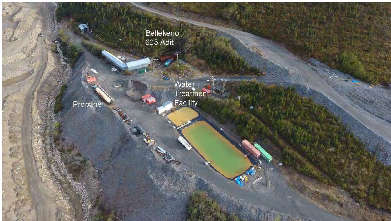
Photo 2-2: Bellekeno 625 Adit Surface Facilities from 2018.
