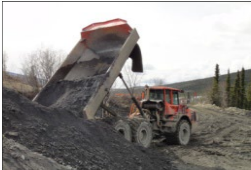
Photo 4-1: Run of Mine (ROM) Coarse Ore Storage
