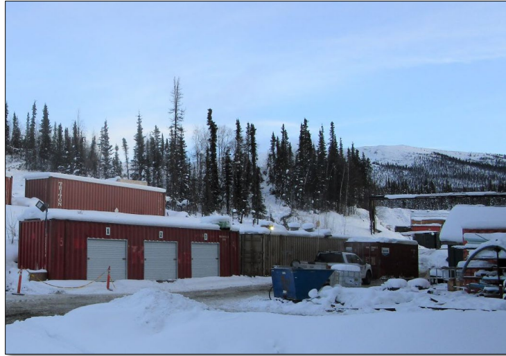
Photo 3-6: Mill Cold Storage
