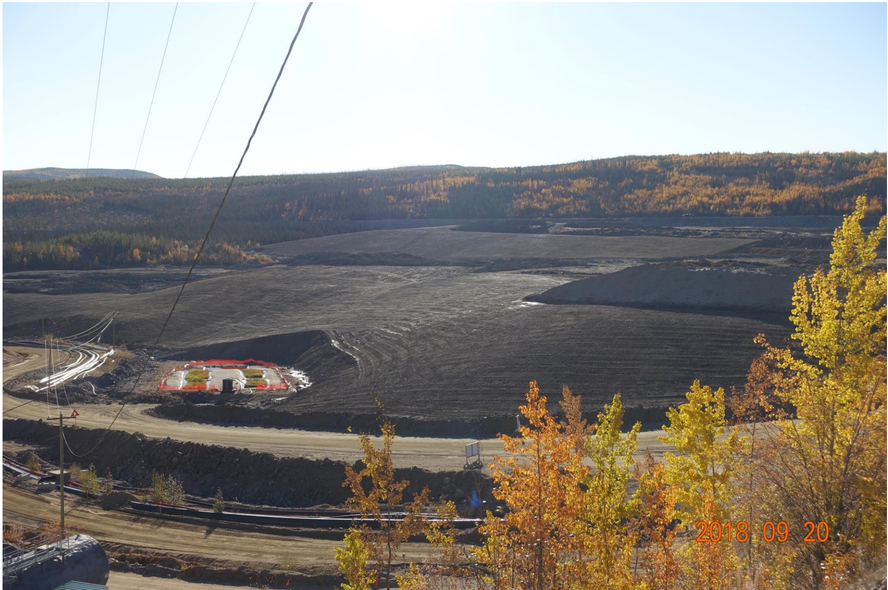
Figure 16-5: MVFE and DST fine grading completed (September 2018)
