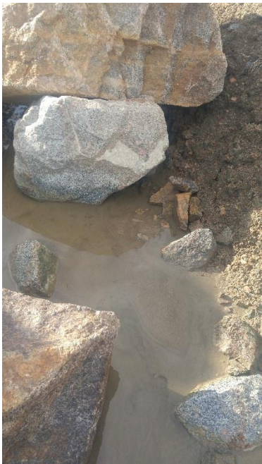
Figure 2-74: SS8 Upstream (Fall 2018)
