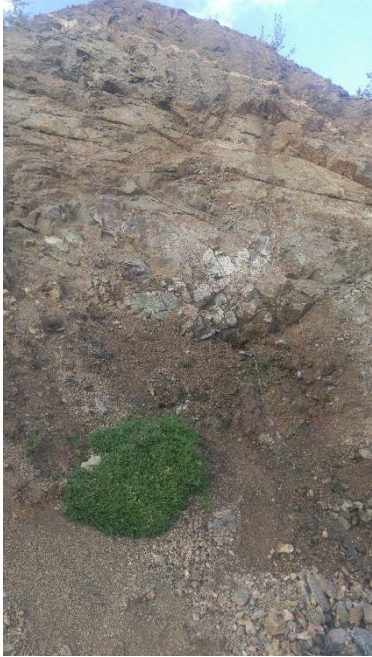
Figure 2-84: SS32 Upstream Rock Face (Fall 2018)
