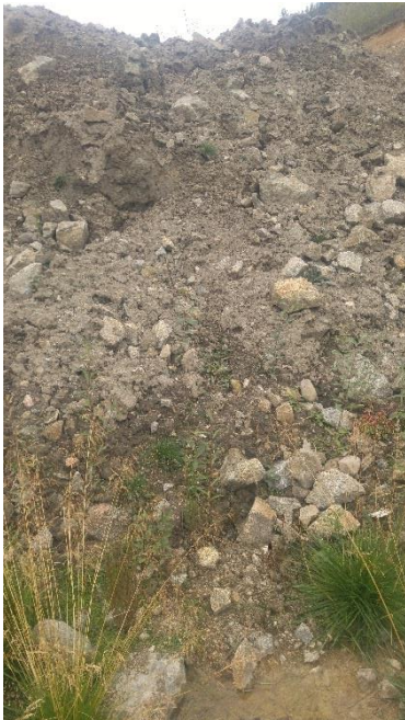
Figure 2-13: SS61 Upstream (Fall 2018)
