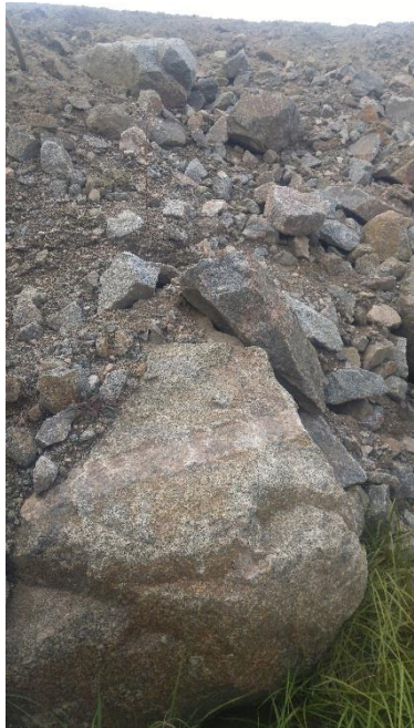
Figure 2-98: SS48 Upstream (Fall 2018)
