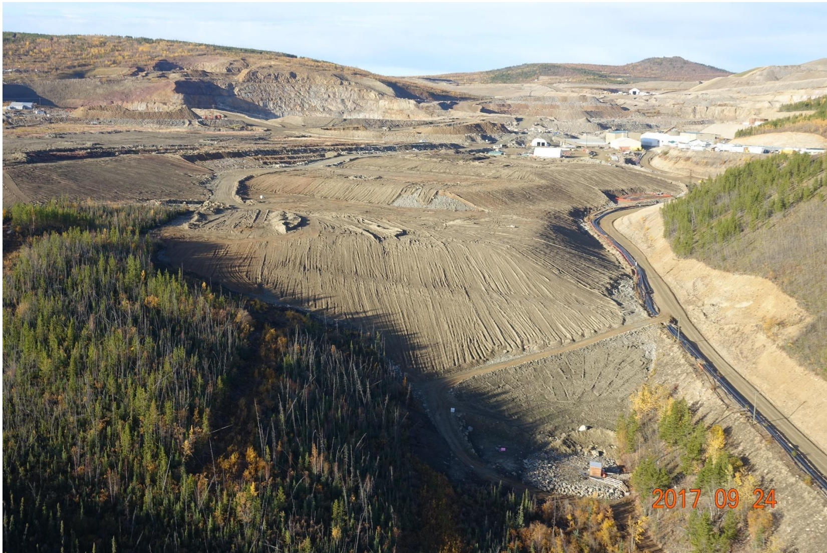
Figure 16-2: Minto Mine – Overburden cover pushed into place on the MVFE and DSTSF (2017).
