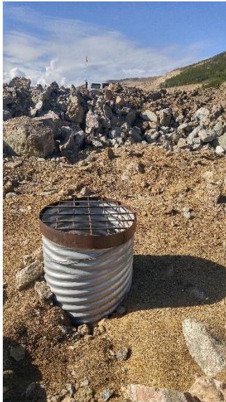
Figure 2-18: W8A Culvert Catchment (Fall 2017)
