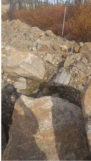
Figure 2-33: SS43 Upstream (Fall 2018)
