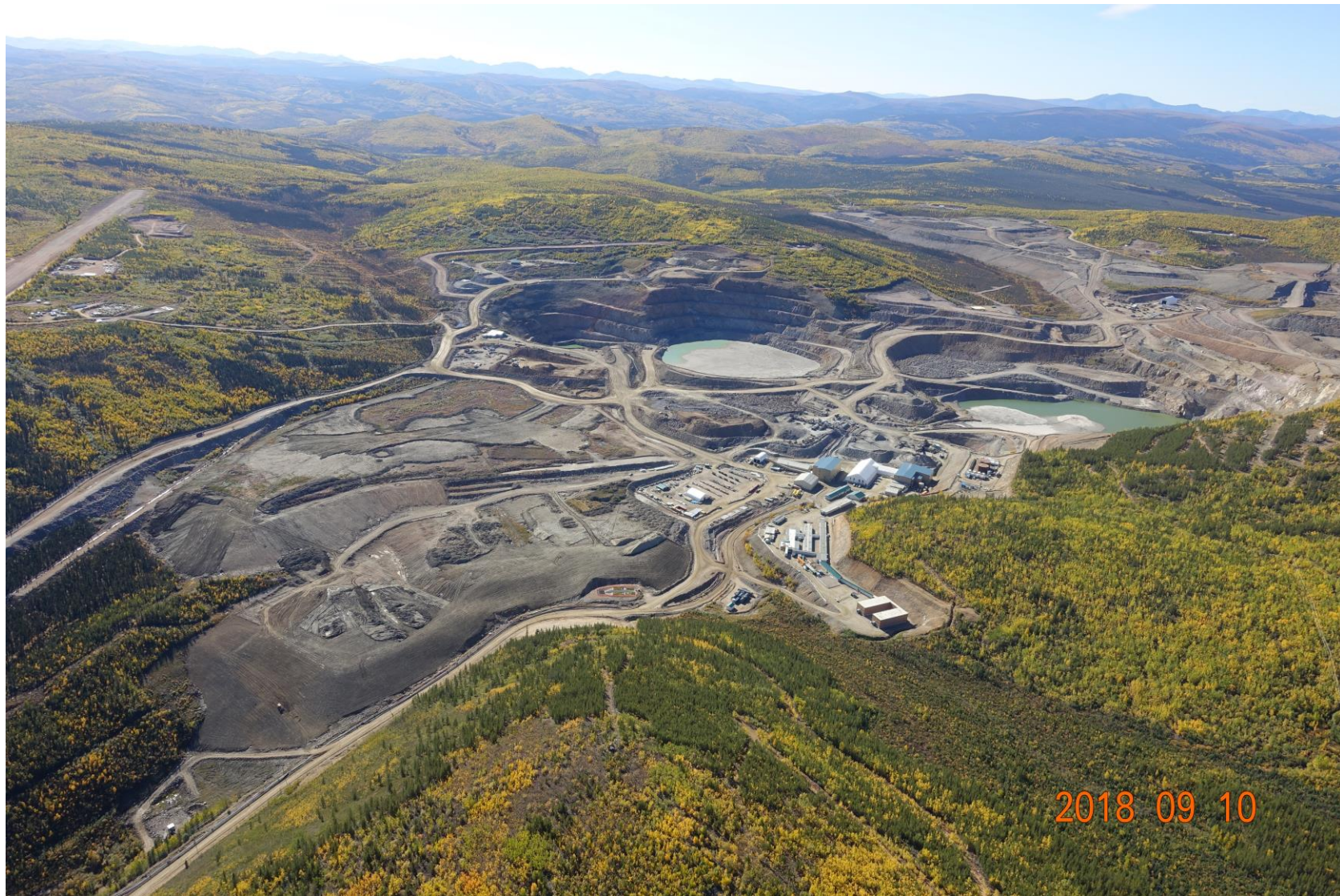
Figure 16-6: Minto Mine – Site overview.
