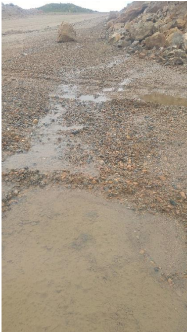
Figure 2-90: SS102 Upstream (Fall 2018)
