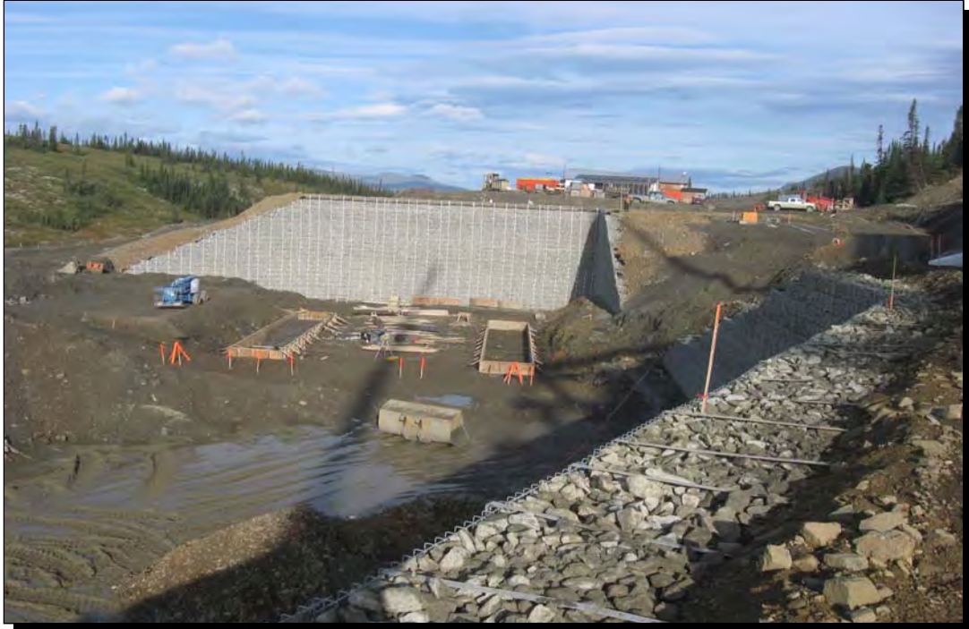
Photo 10 Aug 28, 2009 - Crusher Site and MSE Walls 2A (background) and 2B (foreground) – Looking West
