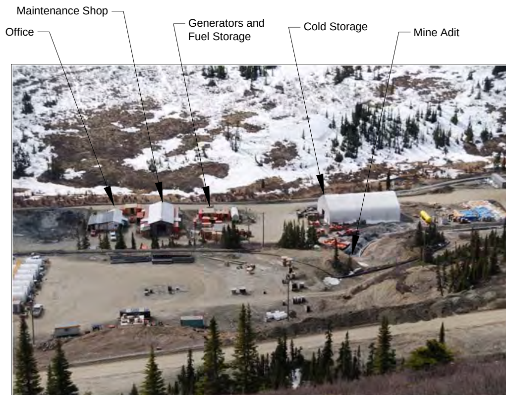
Picture 3-2: Mining Contractor Office, Maintenance Shop and Cold Storage Buildings with Fuel Storage
