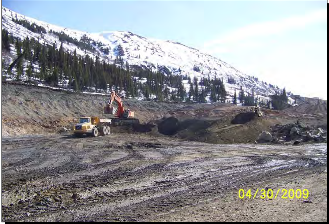
Photo 2 Mill Site Earthworks – Looking East-NE
