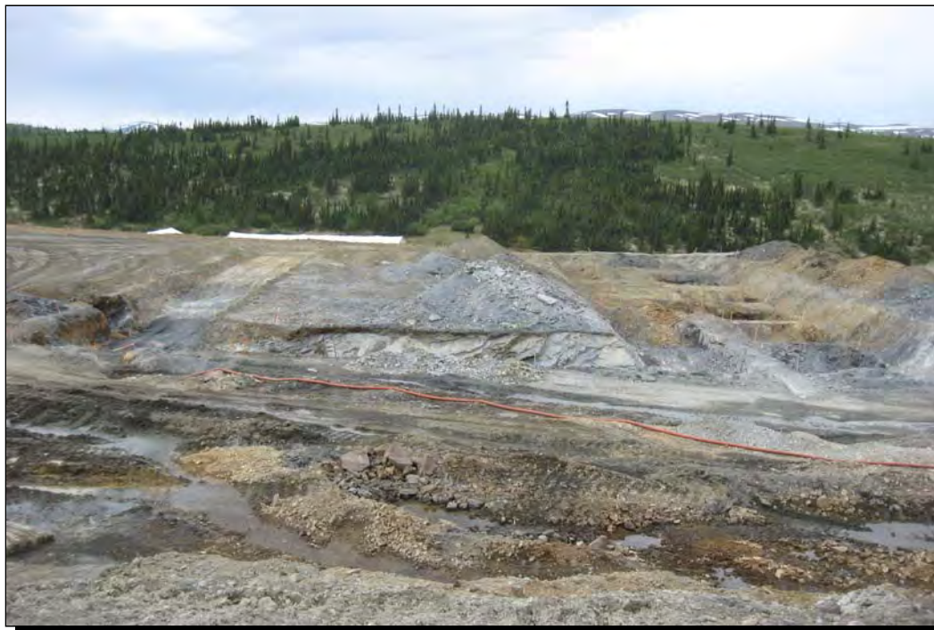
Photo 4 June 20, 2009 - Mill Site – CLO foundation excavation – Looking South
