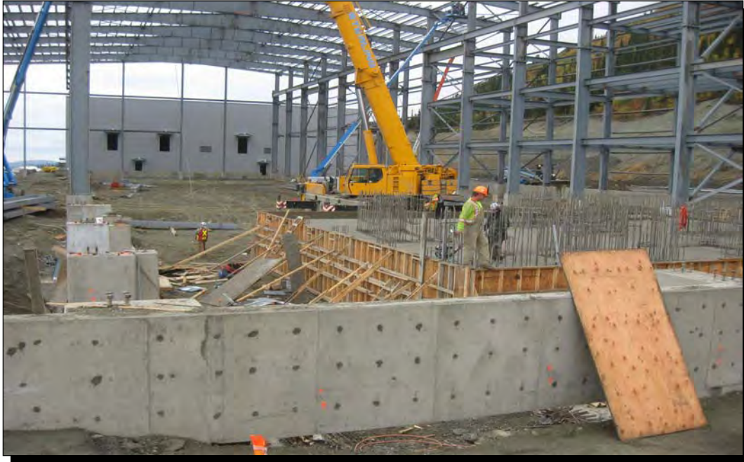
Photo 7 Sept 6, 2009 - Mill Bldg grade beam walls & rod mil foundations – Looking West
