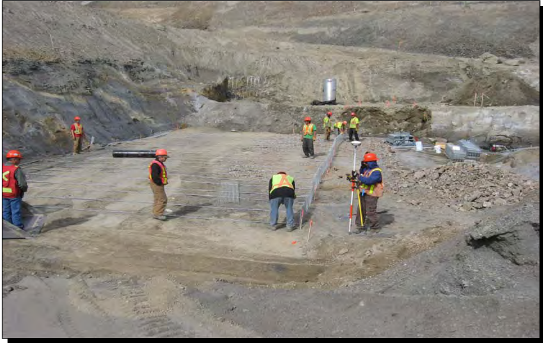
Photo 9 July 24, 2009 - MSE Wall 2A foundation excavation and 1 st Row installation– Looking North
