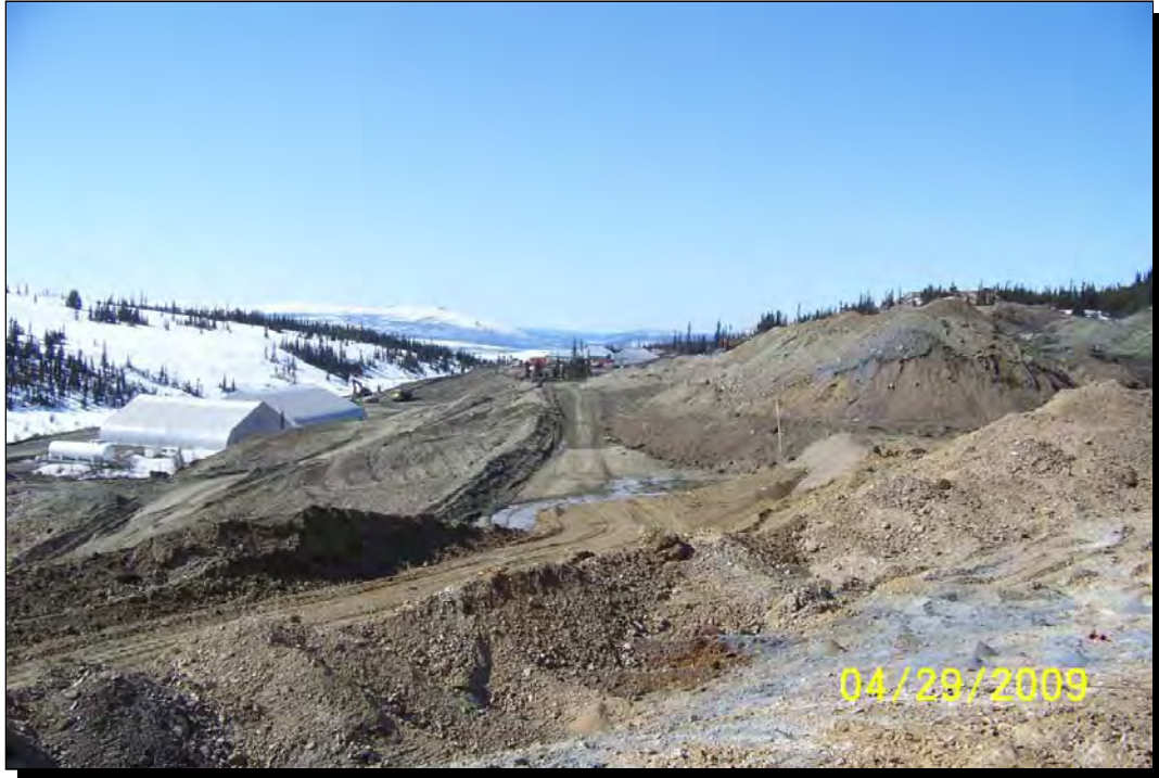
Photo 1 Mill site earthworks – Looking West
