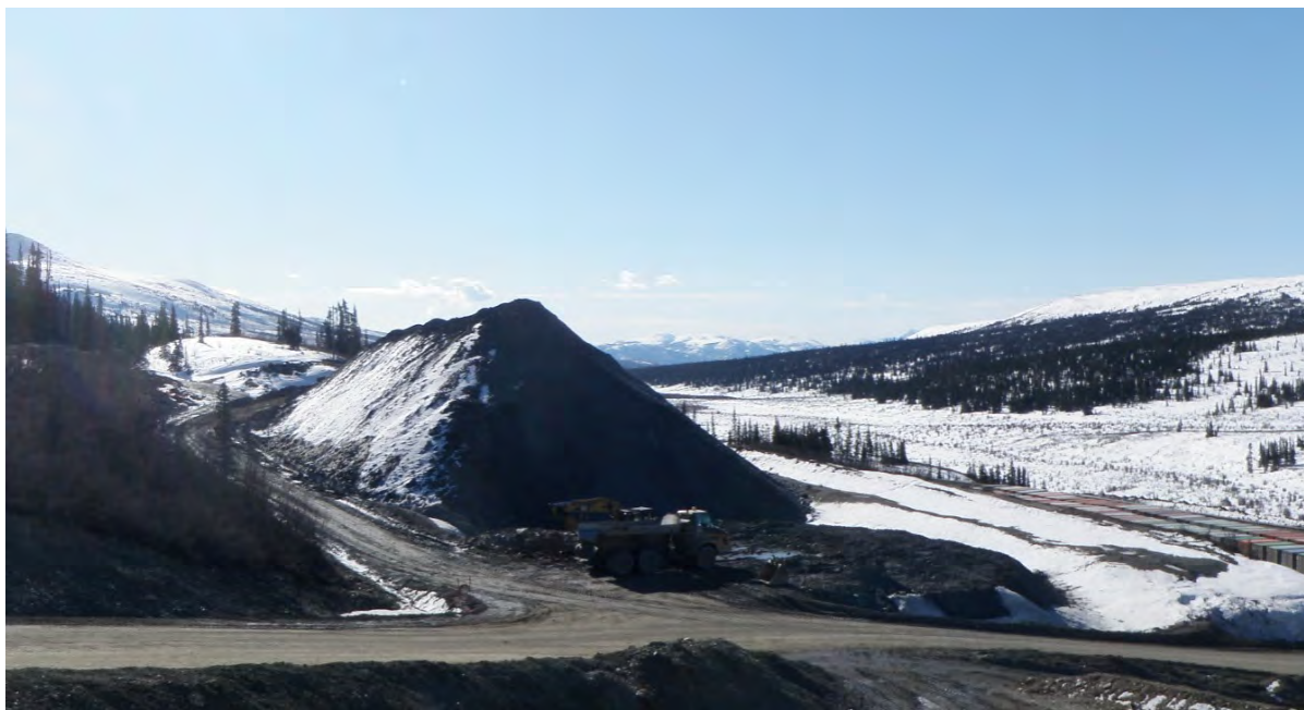
Picture 6-1: Temporary Waste Rock and Ore Storage Facility (April 24, 2010)
