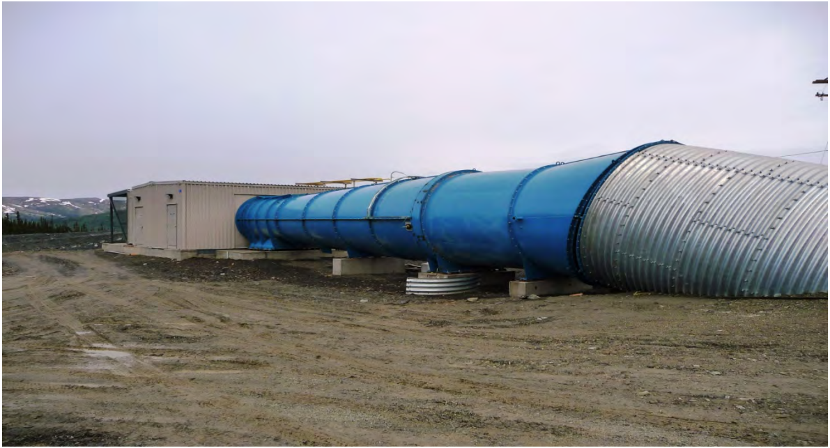
Picture 4-1: Surface Infrastructure – Mine Vent Air Raise (May, 2010)
