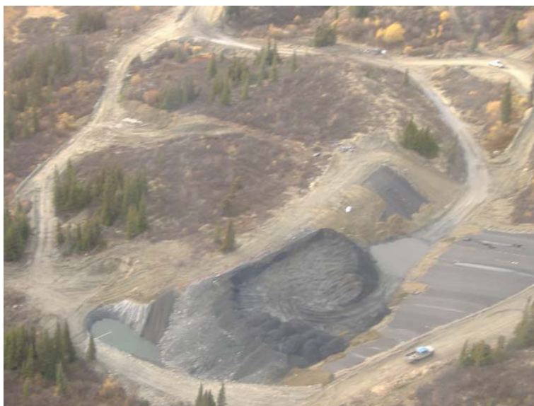
Picture 3.3. Waste Rock Pad and Collection Sump (Sept. 19, 2005)
