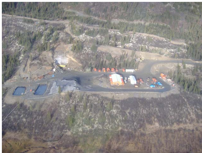
Picture 3.1. Portal Infrastructure (Sept. 19, 2005).
