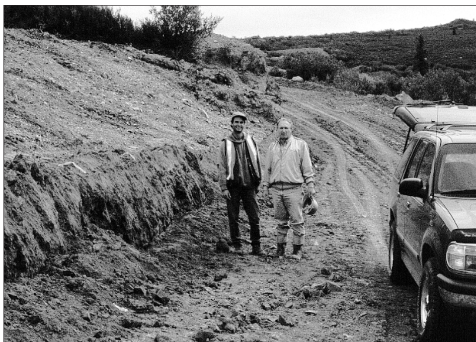
Figure 8. Oxide material exposed by stripping of the Flex zone at the Mt. Nansen Mine. Detailed work for mine planning began on the Flex which is slated for production when the ore from the Brown-McDade pit is depleted.
