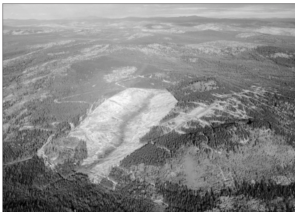
Figure 9. Western Copper Holdings stripped the pad site for the Carmacks Copper Project in 1997. Production of copper from the oxide deposit, using solvent extraction-electrowinning technology, will come from the No.1 zone, marked by trenches at the top right of the cleared pad site.
