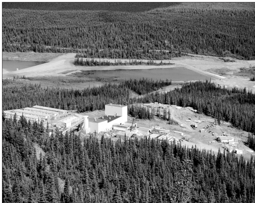
Figure 10. The Sa Dena Hes Mine underwent preparations for a possible reopening. With the right conditions in the zinc market the mine could resume production with short notice.
