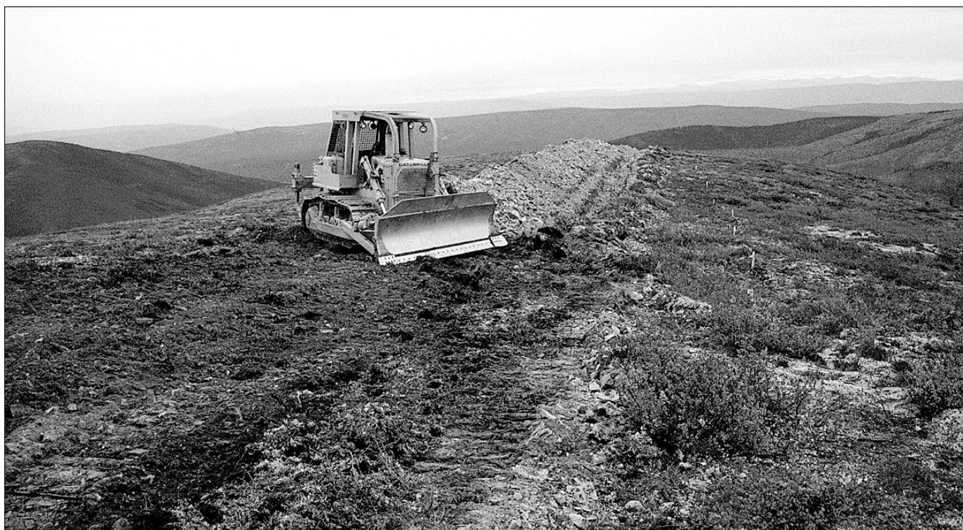
Figure 33. Kennecott Canada conducted an extensive exploration program on the Scheelite Dome property. Trenches excavated during the program were backfilled at the end of the year. La Teko Resources has recently optioned the property and plans more work for 1998.
